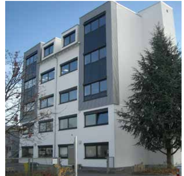
Concept Heidelberg office building in Heidelberg, Germany
